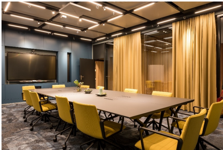
Sennheiser’s TeamConnect Ceiling 2 fits elegantly into the modern appearance of the Mercato conference room
